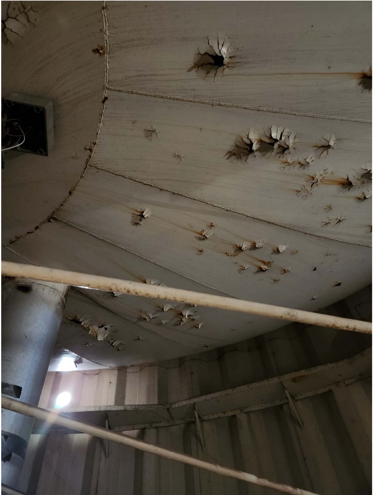
Photo 4 - Interior Dry Bottom of Bowl and Overflow Pipe
