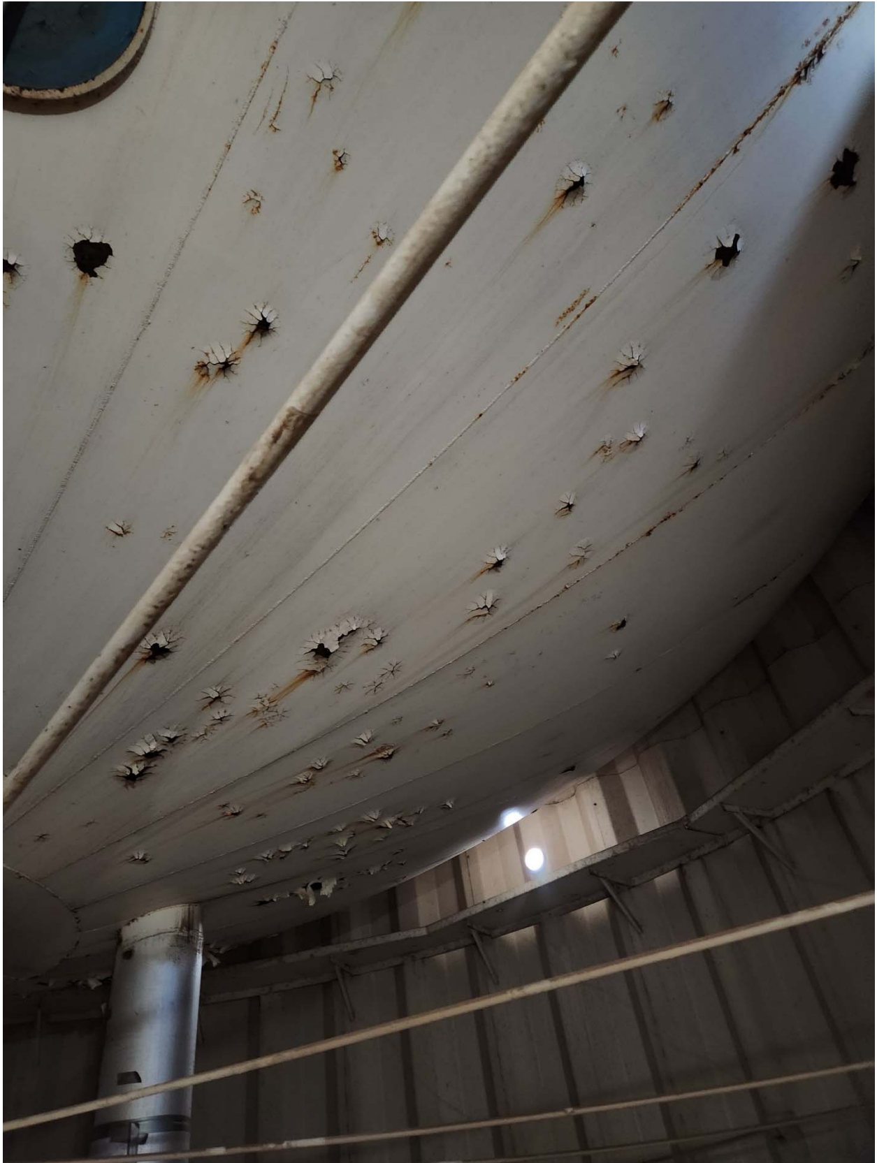
Photo 1 - Interior Dry Bottom of Bowl and Overflow Pipe
